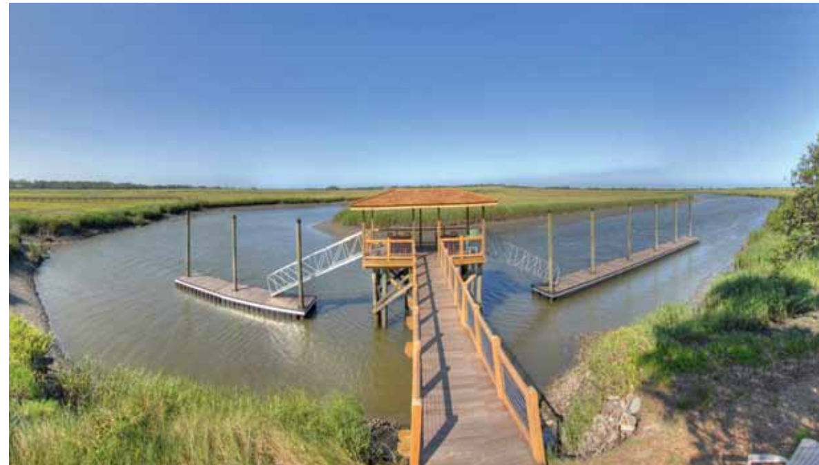
COMMUNITY DOCK WITH 300 FEET OF DOCK SPACE JUST FOR RESIDENTS
